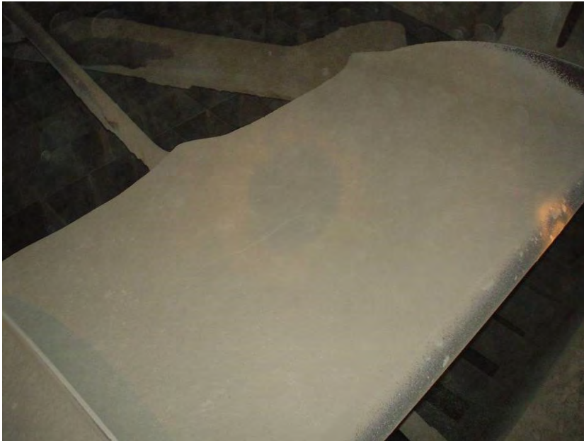
Ash Buildup on Vanes
