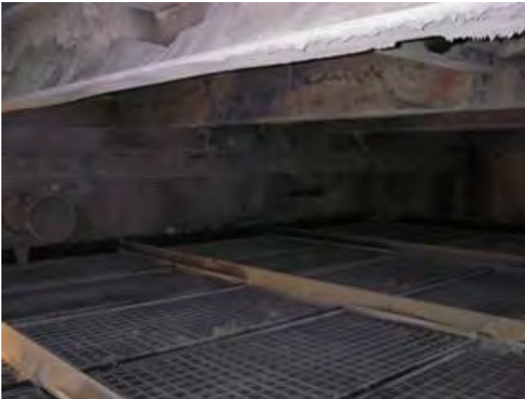
CERAM Cover Grate in Level 1 (Welded Stainless Steel 1 mm Dia. with 5 mm Opening)
