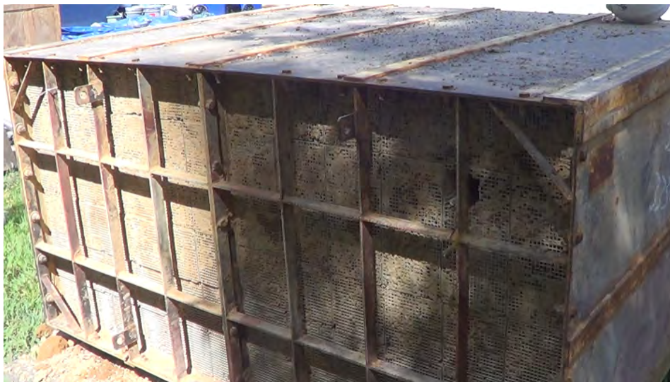
Before Sponge Blasting
