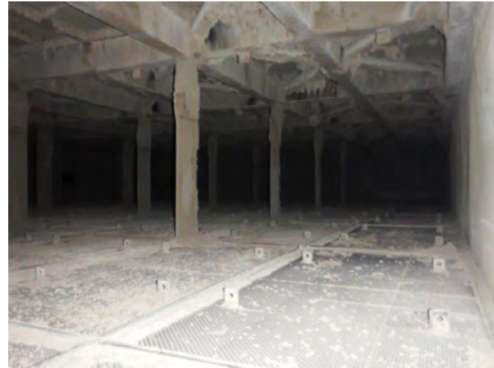
After Install of LPA Screen
